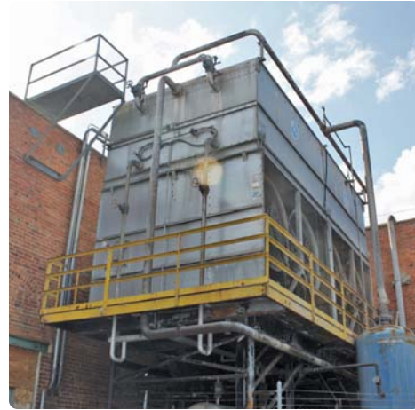
BAC Evaporative Condenser
