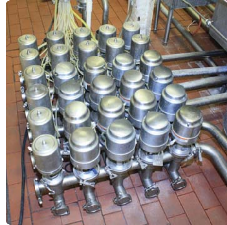
Tri-Clover 30-Valve S/S Air Valve Cluster
