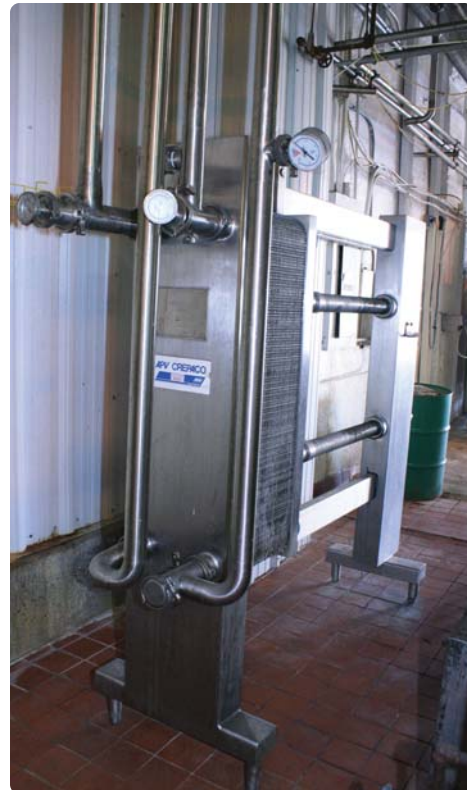
APV Crepaco Plate Press Heat Exchanger
